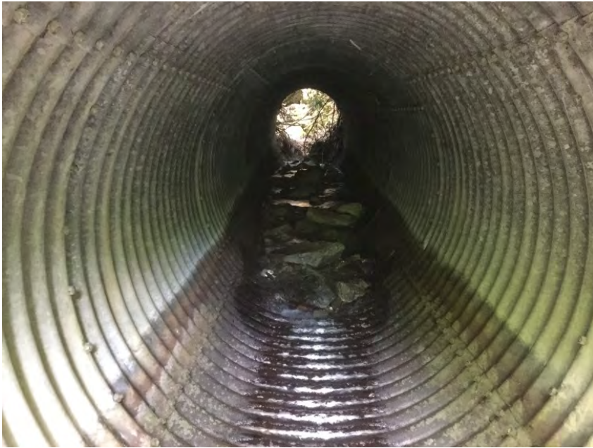
Looking through culvert from outlet
